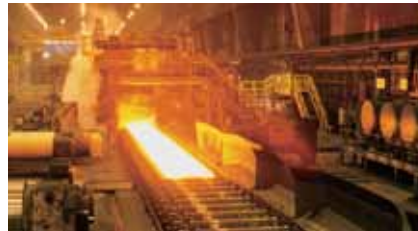
Steel Plant Facilities
